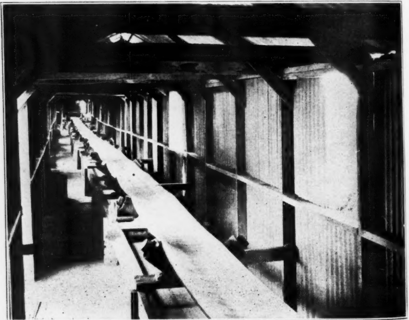
Belt Conveyor to the Loading Bins
